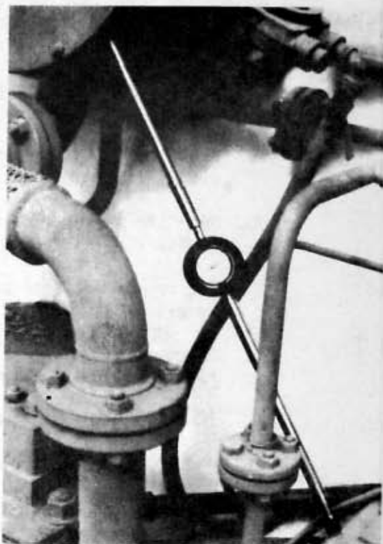
Fig. 4 - Reference measurement being taken between bearing housing and foundation.
